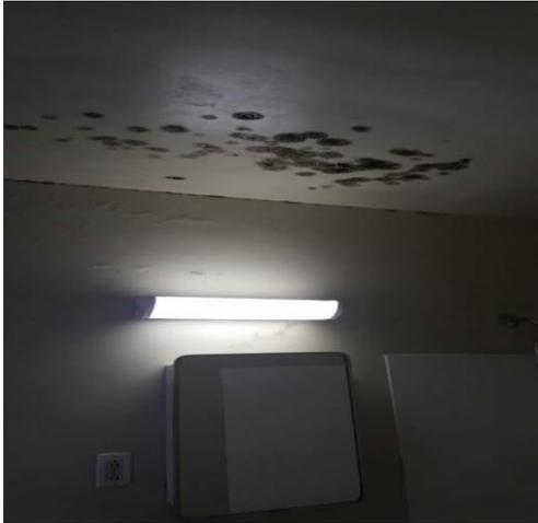
**Carpenters note mold growing through the bathroom dropped ceiling.**
