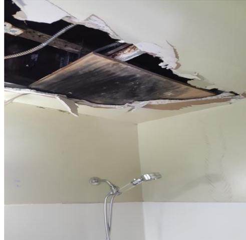
**Photo of ceiling sheetrock removed. Mold is visible on the wood frame above the ceiling.**
