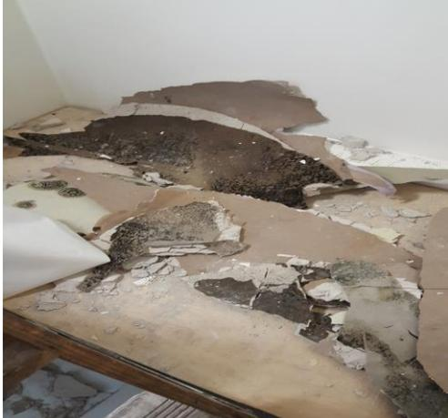
**Photo of the top side of the sheetrock removed by Carpenters. It is infested with mold from the wood frame area.**
